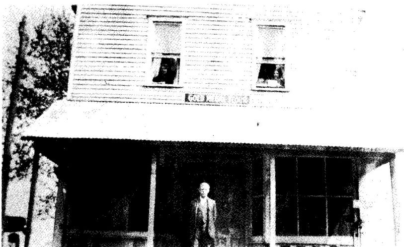
An old snapshot of country store at Motor, Iowa. Concluding event in this installment occurred on front steps of this store.
